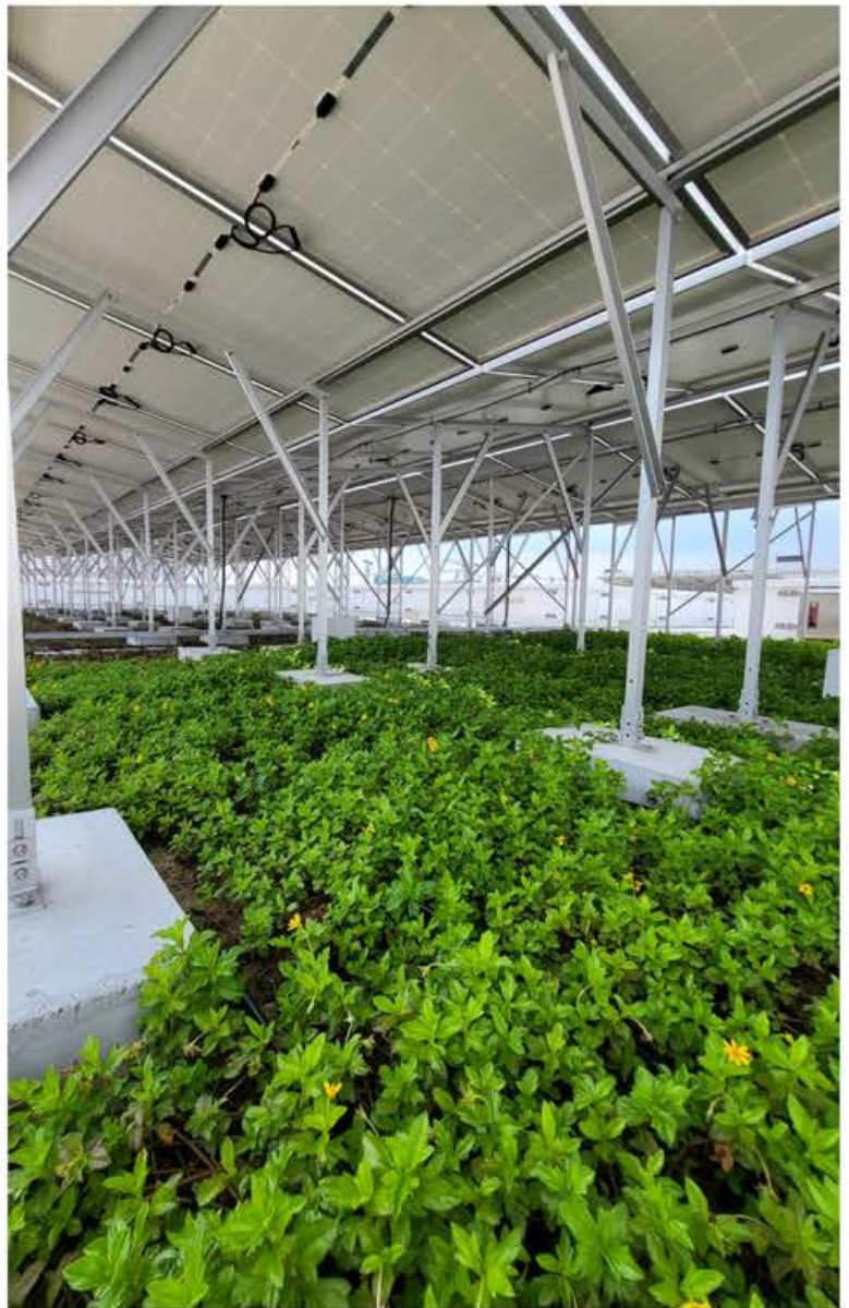
Plant selection has to be done carefully to ensure that the plants not only thrive well under the solar panels, but do not interfere with the capturing of the solar energy.
